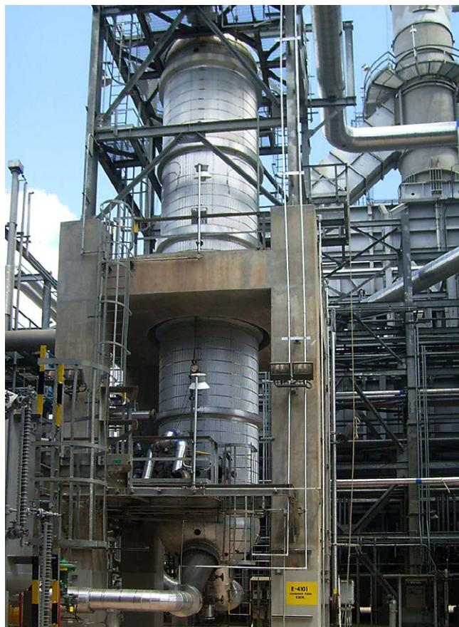
Packinox heat exchanger installed in a catalytic reforming unit.
