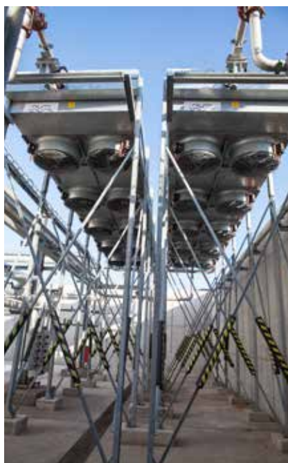
Two Alfa Laval ACHEs (Air-Cooled Heat Exchanger) provide effective cooling of the cooling medium.
